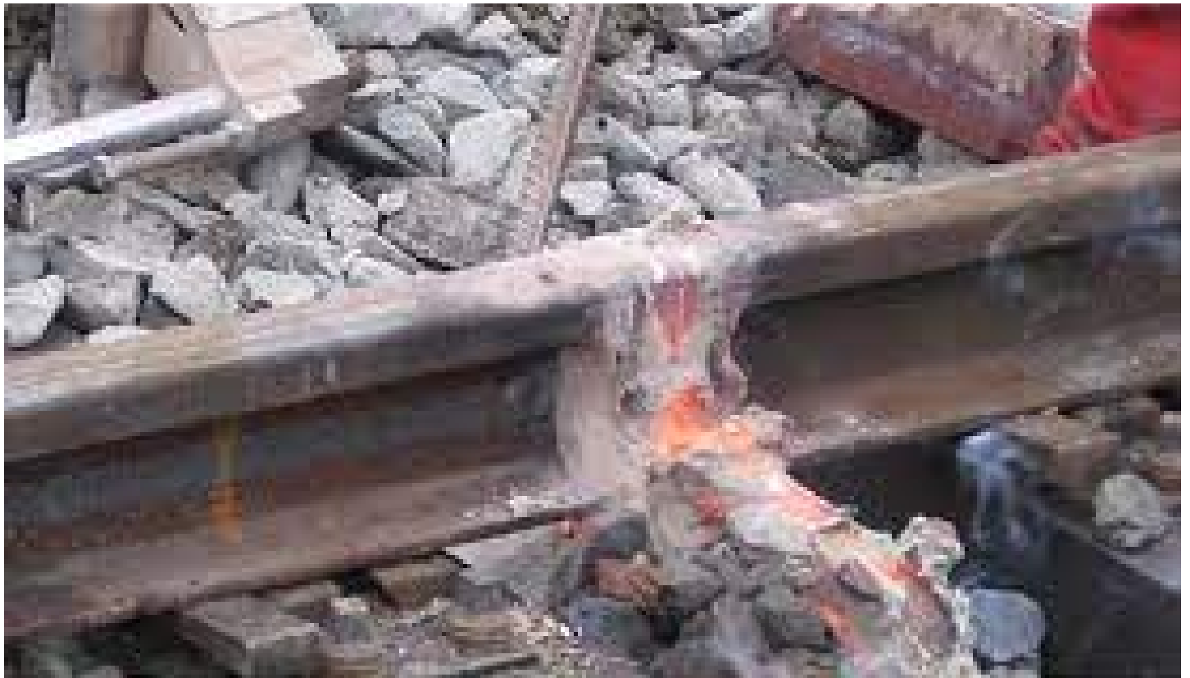
Thermit Welding on Railway Track
