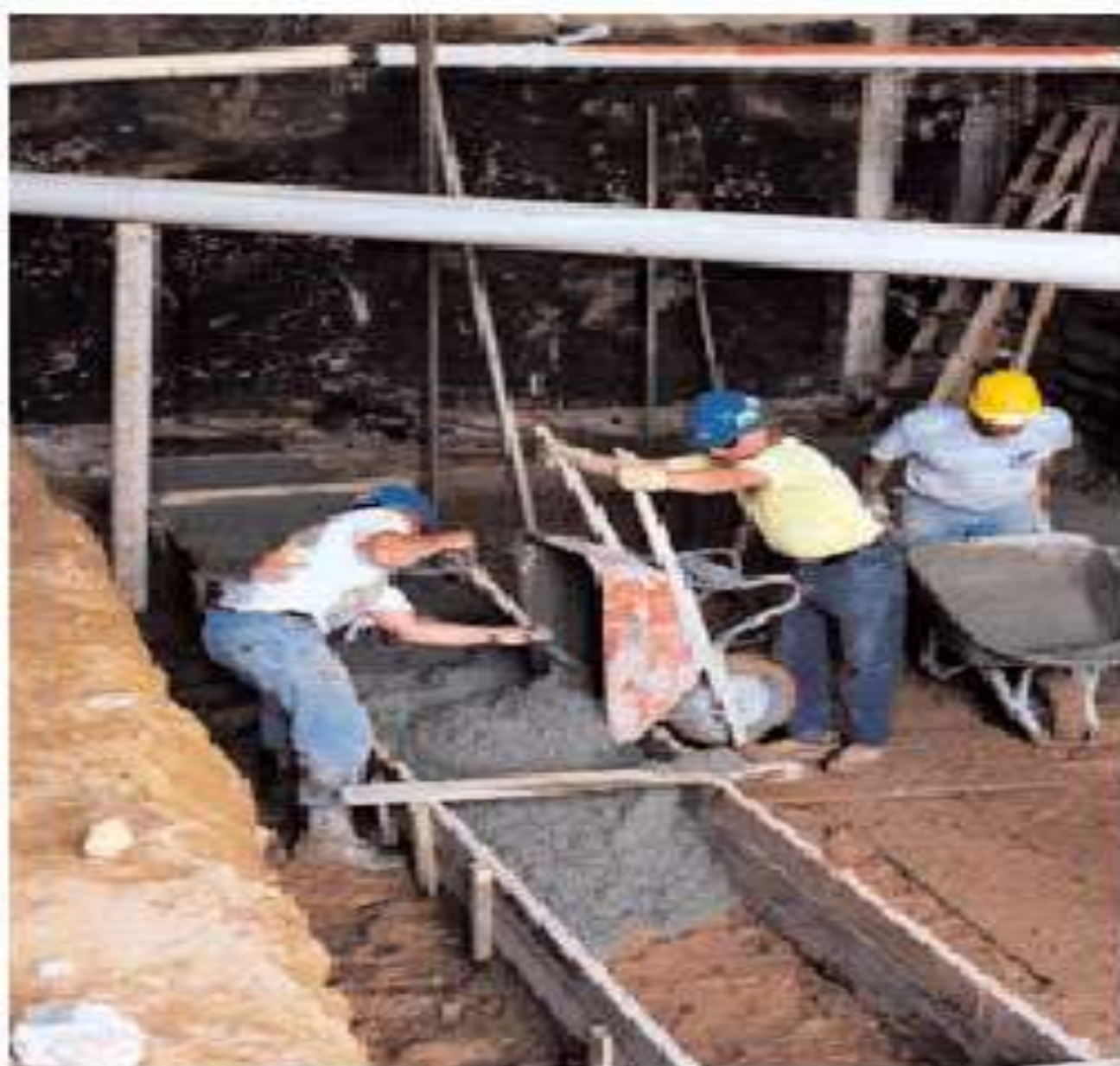
Fig. 11-4. Wheelbarrows are used to place concrete in areas that are not easily accessed by other placement methods. (69929)
