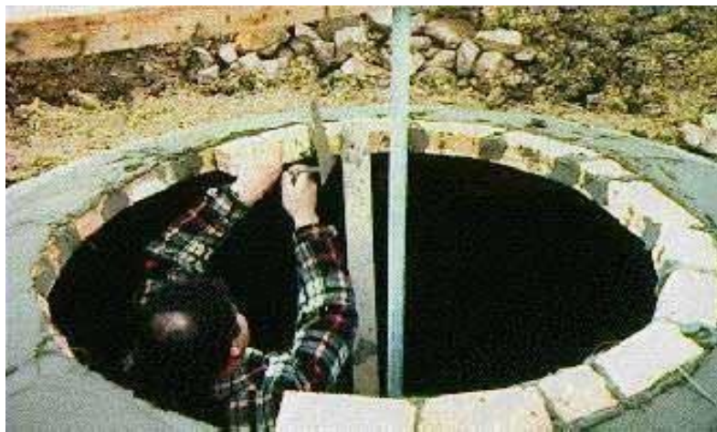
Figure3:Fixed-domeplantinTunisia.Thefinallayersofthemasonry structure arebeingfixed.
