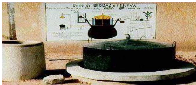
Figure 7: Floating-drum plant in Mauretania
