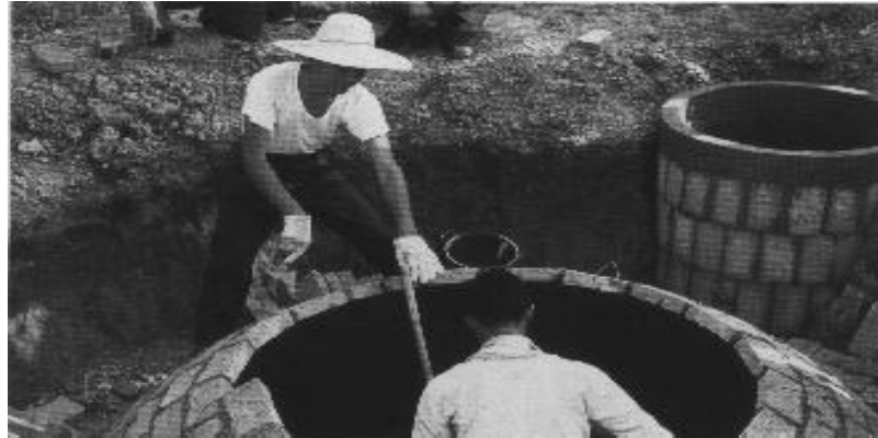
Figure 6: Installation of a Shanghai fixed-dome system near Shanghai, P.R. China
